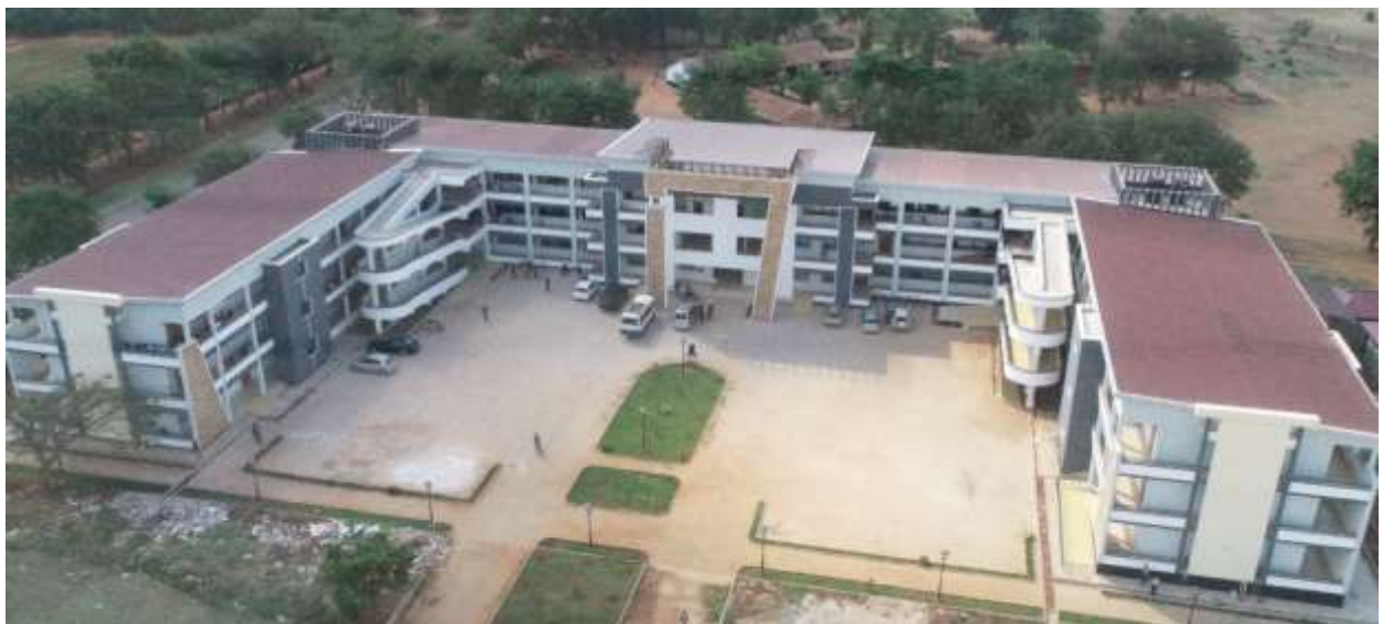
Newly constructed Multi-Purpose Laboratory infrastructure at the Edward Moringe Campus
